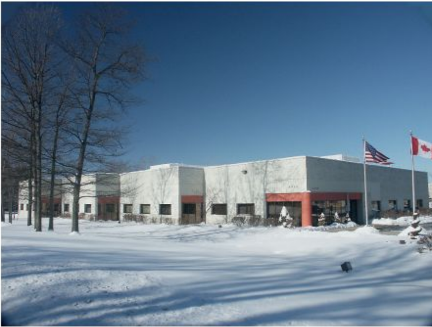
Industrial - Small Factory in Troy, Michigan
