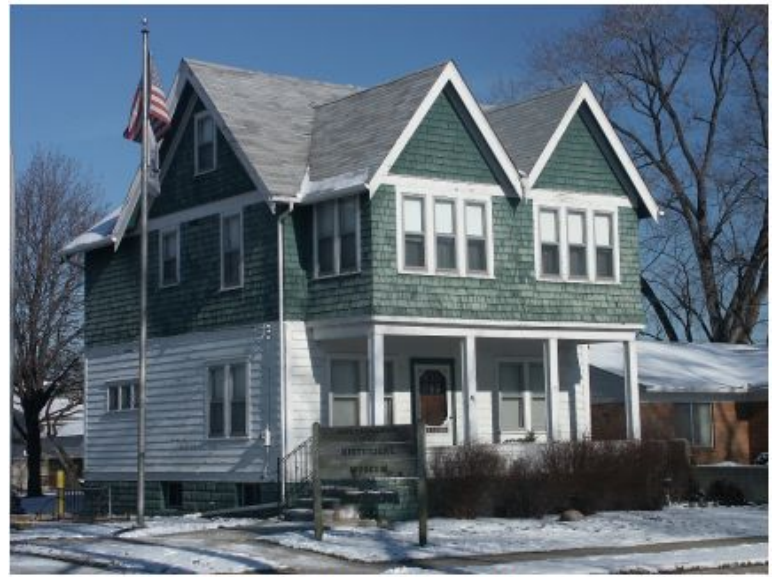
Preservation of a House - Clawson Historical Society (Museum That Needs Restoration)
