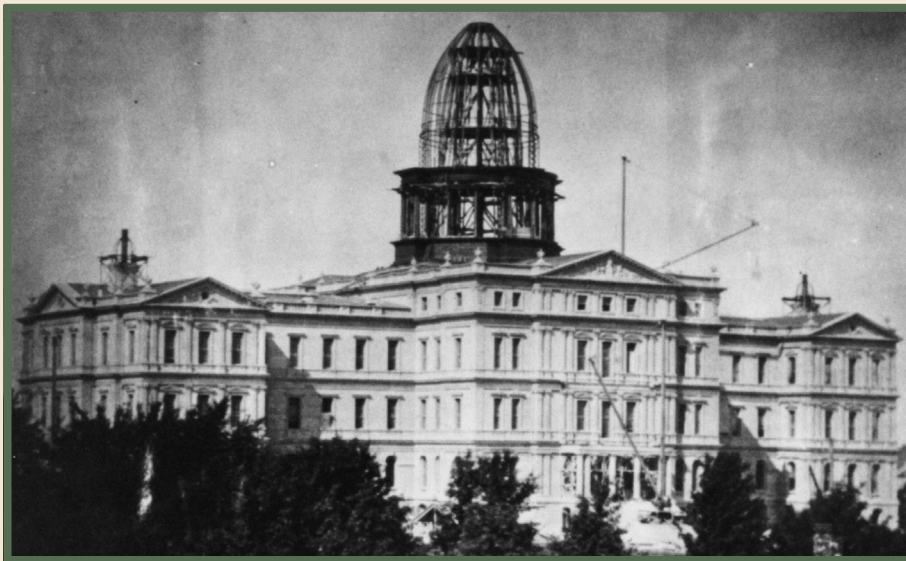
Made of wrought and cast iron from the S. J. Creswell Ironworks in Philadelphia, the dome took almost a year to build. (Image courtesy of the Archives of Michigan)
